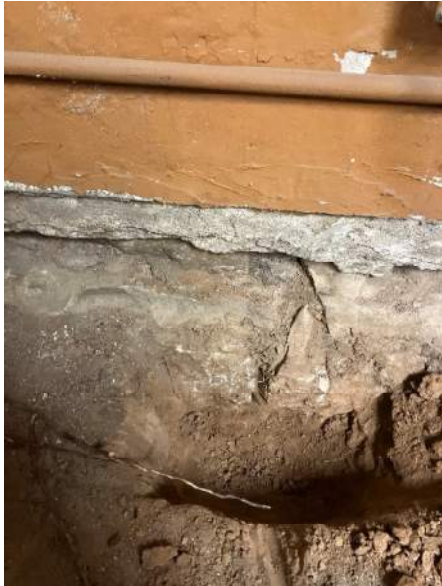
Exposed Foundation Stone
