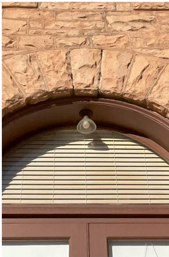
Photo #15: Exterior lighting over door
