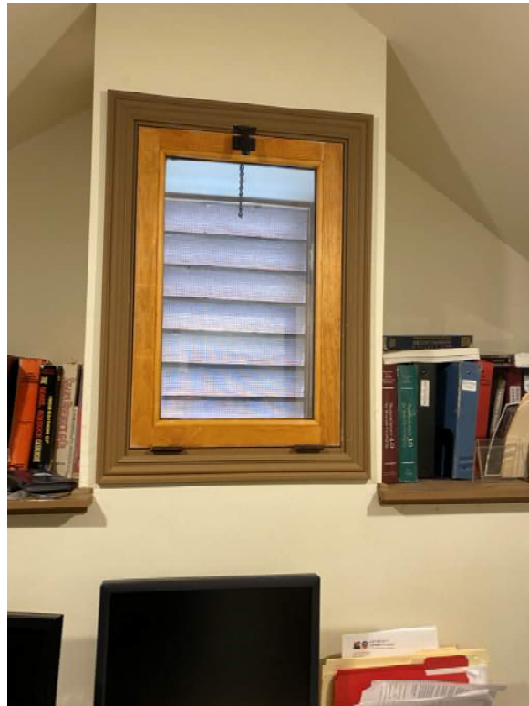
Window in Attic Office
