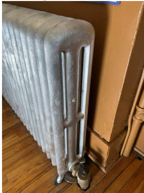
Typical Radiator and Manual Control Valve
