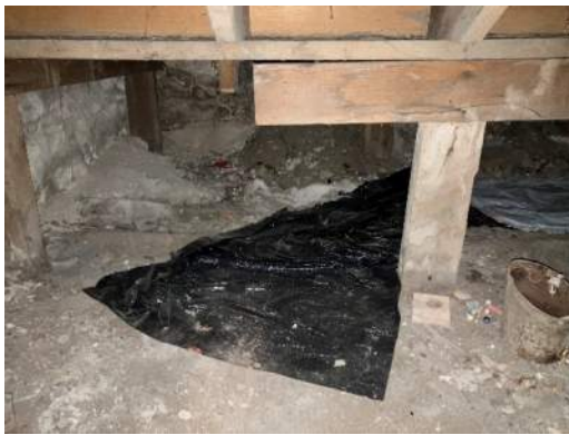
Support at Lower Stair Landing
