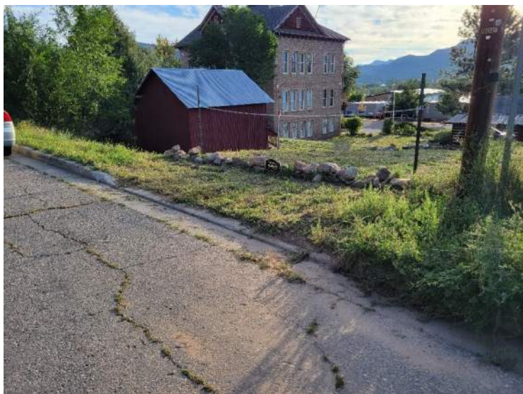
Figure 2 - West 3rd Avenue driveway
