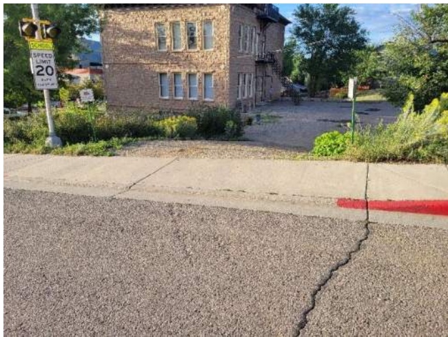
Figure 1 – Existing 31 st street driveway access
